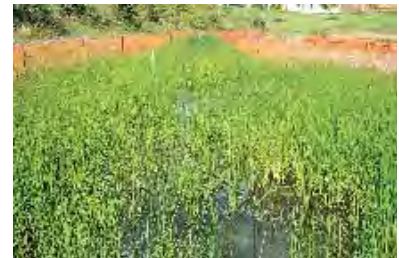
A wetland mitigation project under construction. When wetlands are impacted due to construction, wetland mitigation is required.
