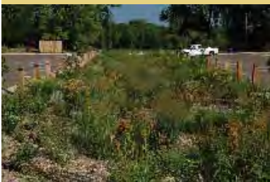
After construction, parking lot runoff is collected in an attractive rainwater garden that infiltrates stormwater.
