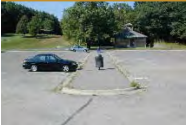
Before construction of the Lone Lake infiltration project, rainwater ran off the impervious parking lot.
