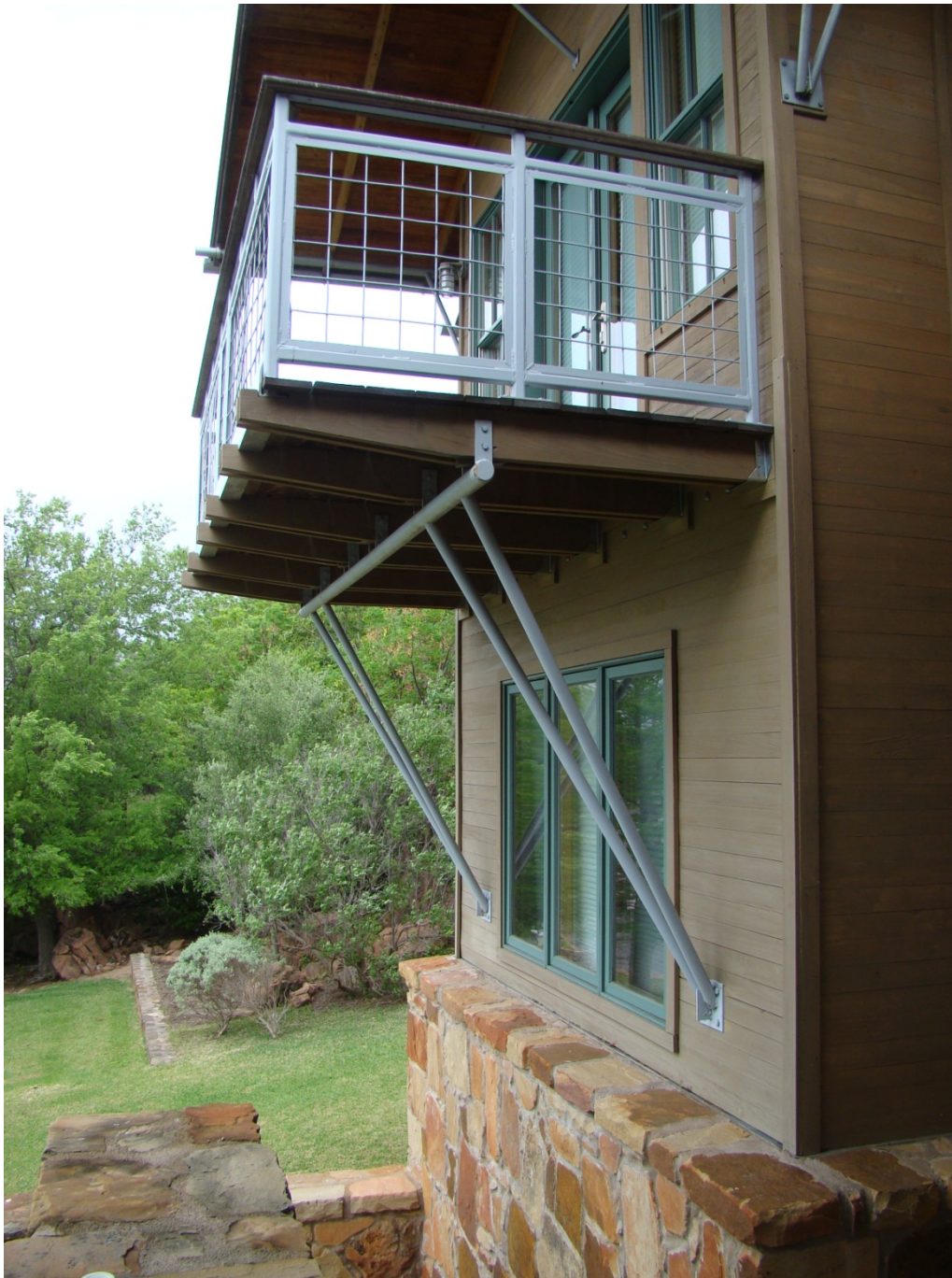
This photograph was taken after the balcony was repaired.
